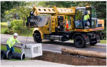
remove the old pipe, and then clean up the ditch. The boom then was used to position three sections of new plastic pipe in the ditch, where one end was attached to an existing drain pipe. Next, the Gradall carefully excavated a place to install a new catch basin, and lowered it into position at the other end of the pipe.
