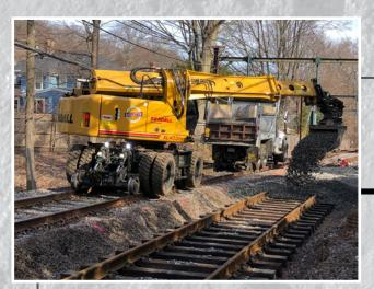
New rail ties and 40-foot sections of continuous welded rail were carefully placed into position before ballast was evenly
