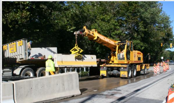
Route 29 in the village of Palm, where a bridge replacement project was under way, the Interstate crew was setting 200 feet of 42-inch barriers, each weighing 9,200 pounds. At each end of the line of barriers were several crash attenuators, each 25 feet in length and weighing about 2,500 pounds. ❖ Blocking off one lane of the two-lane bridge, barriers were set using chains as well as a barrier handling attachment. During the process, operator Joe Bernick repositioned the
