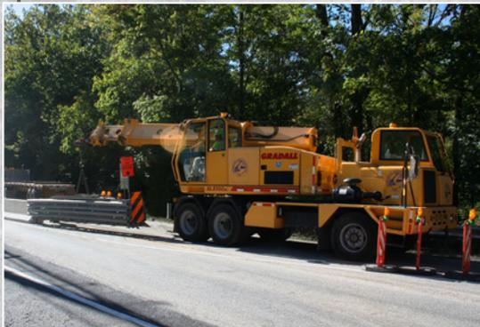
carrier from the operator cab, removing barriers and attenuators from a flatbed trailer and then moving up and down the length of the job site, aligning barriers from inside the job perimeter. Because of the Gradall excavator’s short tail swing, one lane of traffic flow could continue on the bridge while the barriers were being placed.
